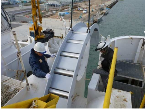
Photo 6: Fitting of replaceable chute
