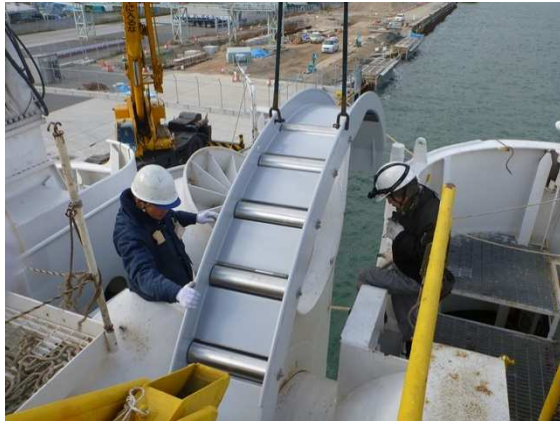
Photo 6: Fitting of replaceable chute
