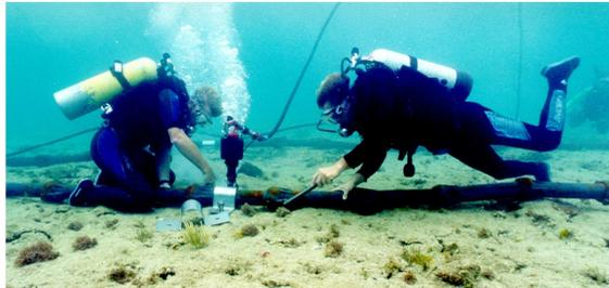
**Figure 5: Clamping Articulated Pipe**
