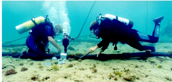
Figure 5: Clamping Articulated Pipe
