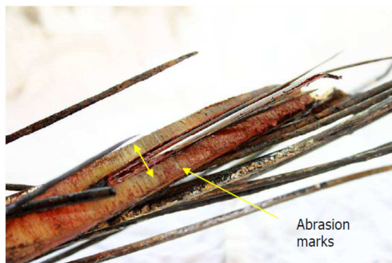
Figure 1: Example of Abraded Cable
