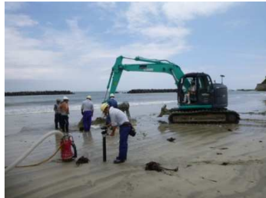
Fig. 8: Existing Cable Localization
