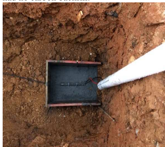
Figure 2 Carbon backfill for sample#3
